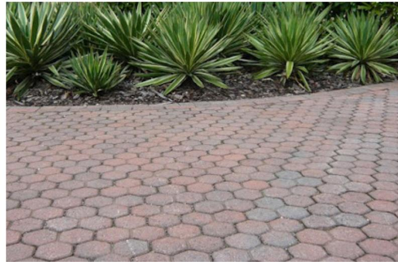
Permeable paving surfaces
