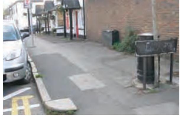
Figure 17 Poor quality paving surfaces, top end High Street
