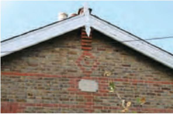
Figure 36 Timber finials and moulded barge boards
