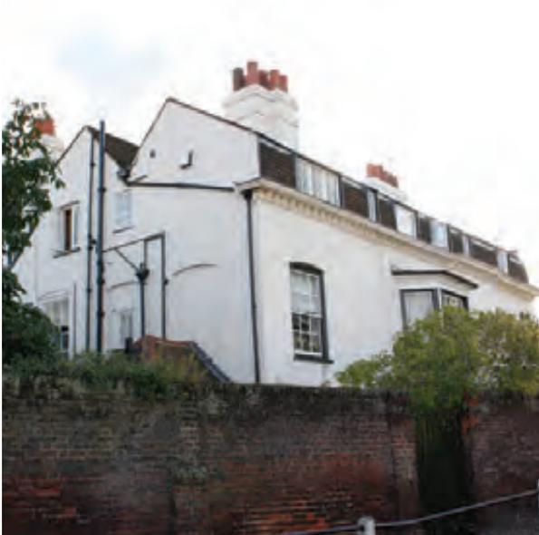
Figure 56 Mansard roof, nos. 1-5 Station Road
