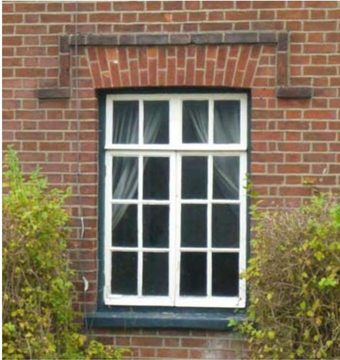
Figure 17: The notable use of bricks to form a hood mould to windows (to Estate cottages)
