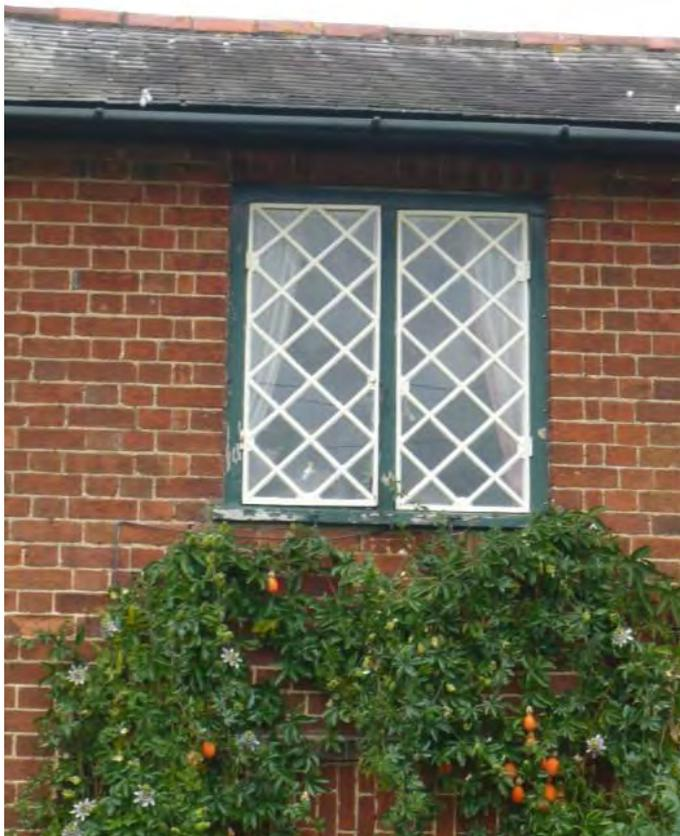
Figure 18: Cast iron casement windows with diamond pattern glazing bars
