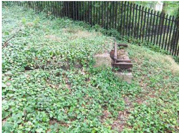
Remains of concrete footings and iron framing from former pedestrian bridge (timber) spanning the Campbell Circuit
