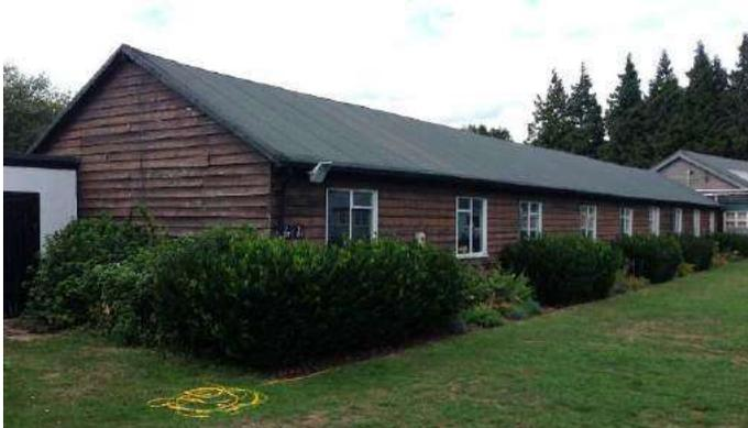
South and east elevations, demonstrating the risks that may arise as a result of vegetation growing against the timber clad walls.
