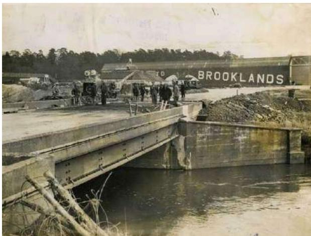
Construction of the Campbell Circuit showing the c.1927 Vickers constructed bridge that was modified to accommodate the new circuit (1936)
