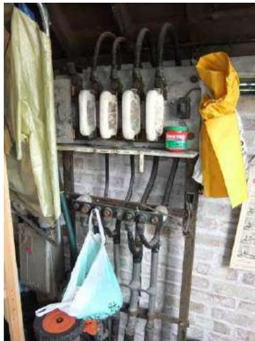
Internal view of the substation, with the original ceramic fuses still in-situ
