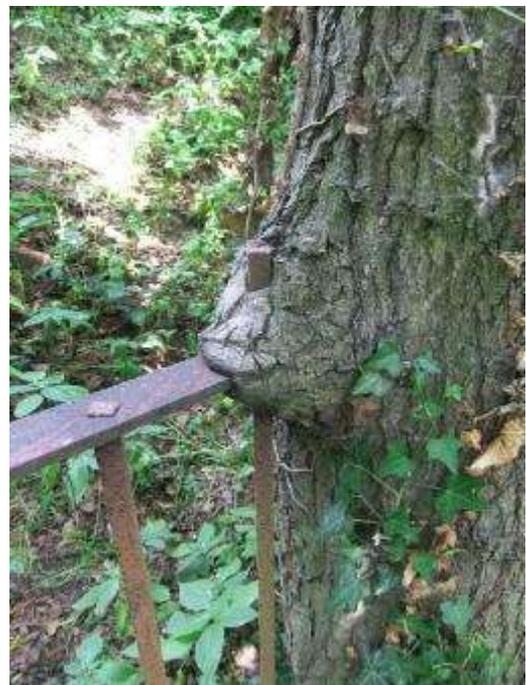
Fig 5.80 - Sections of railings being consumed by the growth of the trees along the support banking.
