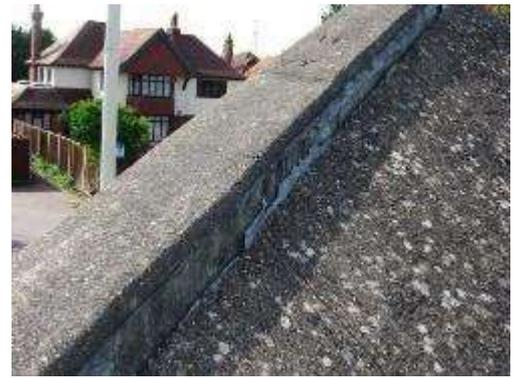
Fig 5.106 - Failed mastic type sealant at the abutment of the former track edge and the retaining wall to Barnes Wallis Drive, clear evidence of movement in the track surface.
