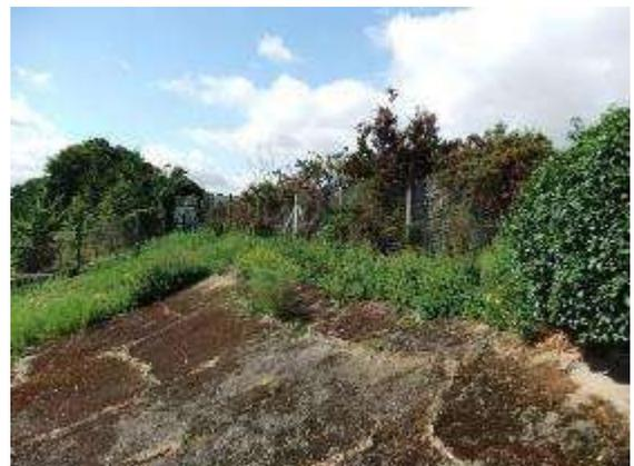
Fig 5.116 - Unmanaged vegetation, weed growth and mosses established around and across the surface of track.
