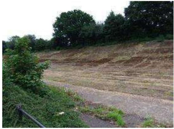
Fig 5.100 - Encroaching vegetation to the lower and top edges of the rack track, and further scars of inappropriate interventions by utility companies along the lower edge.
