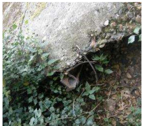
Fig 5.102 - Previous attempts to provide support to the undermined sections of banking, using metal posts.
