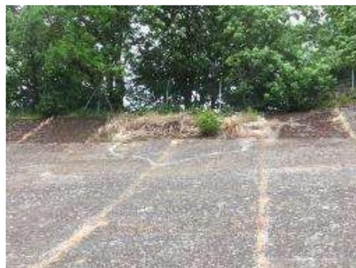
Fig 5.7– Vegetation and weed growth becoming established to areas of track degradation.
