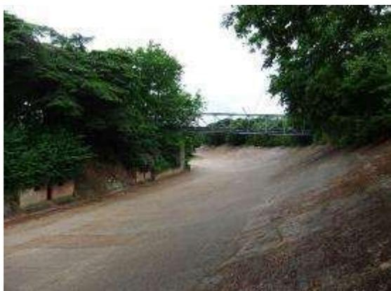
Fig 5.12 – Members' Banking to the north-east side of Members' Hill. Air raid shelters built into the Hill and the scar in the track surface showing the late-twentieth century repairs in the location of the former hangar.
