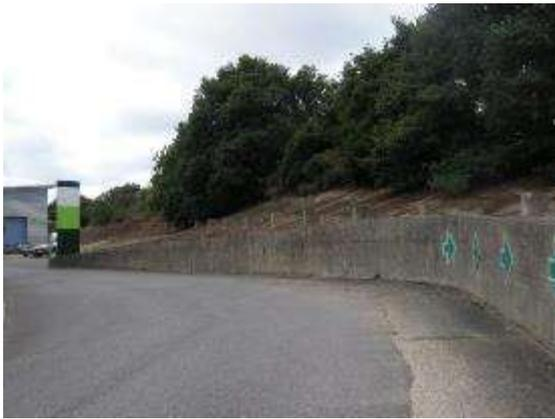
Fig 5.111 - Inner edge of the track, lost when BAC built new industrial facilities here in the early 1960s. Concrete bases supported services to this area of the aircraft factory.
