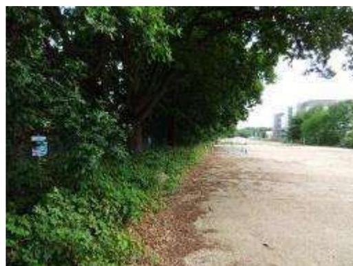
Fig 5.43 - Vegetation encroaching across the track obscuring and potentially destroying the original edge treatments and alignment.
