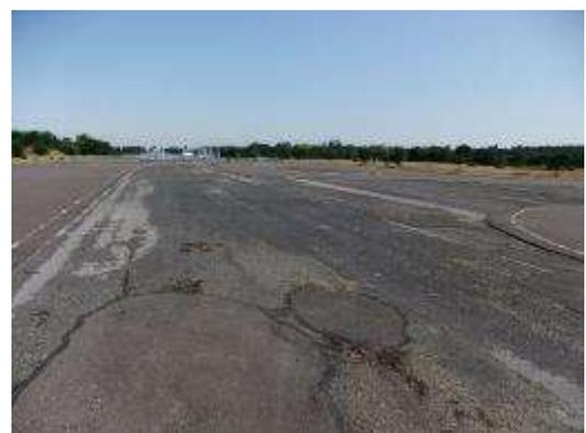
Fig 5.86 - Sections of the runway surface remain exposed in the locations of a former go-kart track.
