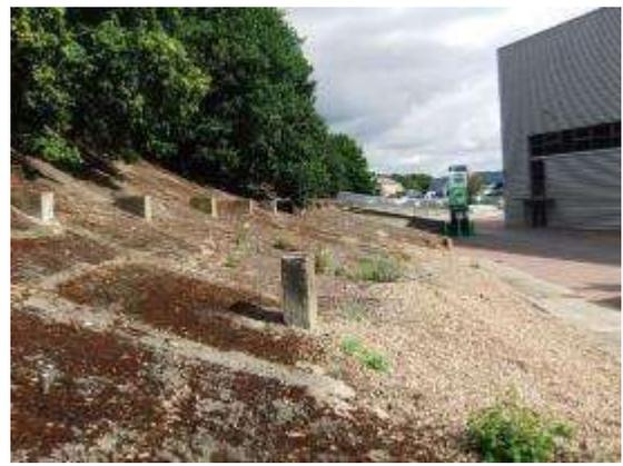
Fig 5.112 - Gravel has been laid over a geotextile membrane in the location of the lost inner edge to the track.
