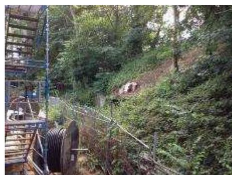
Fig 5.2 – Support banking to the Members' Banking overgrown with vegetation.
