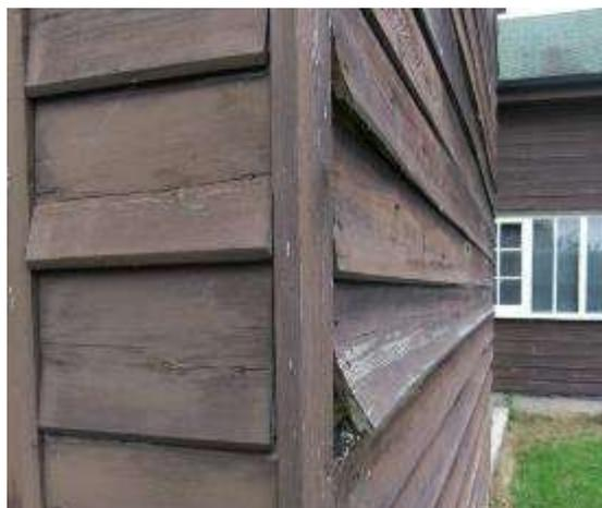
Fig 5.29 – Examples of cupping and distortion to inappropriate replacement weatherboarding on the west side of the Jackson Shed.
