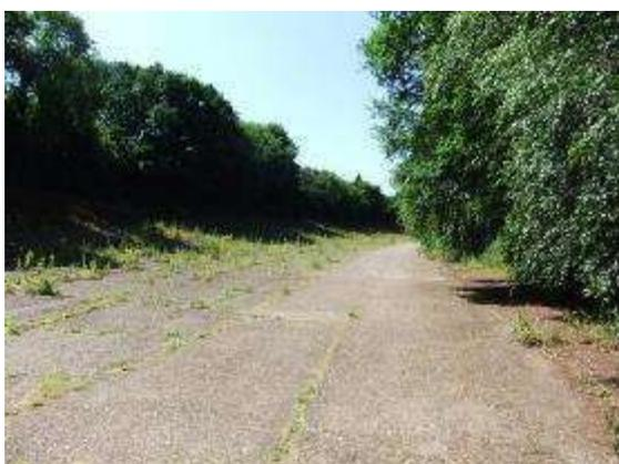
Fig 5.73 - Curving section of Byfleet Banking with the concrete bays clearly identifiable.
