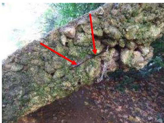
Fig 5.74 - Evidence of bar reinforcement to the now unsupported top of the banked track (southern end).
