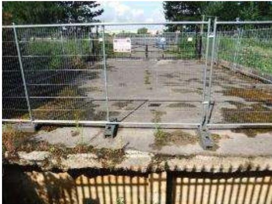
Fig 5.57 – The remains of the former Campbell Circuit Bridge spanning the River Wey. A section of concrete surface to the east side was removed and temporary fencing erected c.2011.
