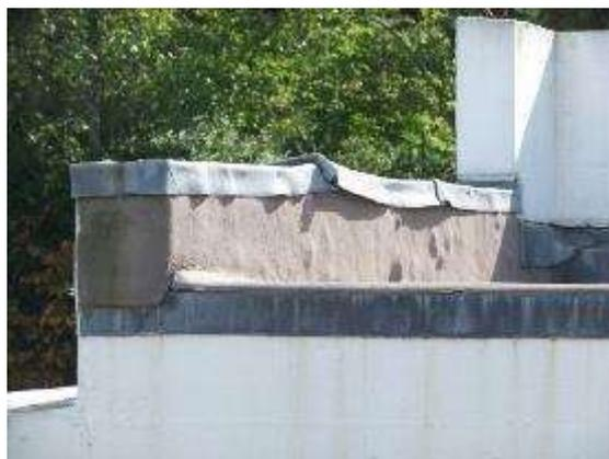
Fig 5.64 – Lead coping to north parapet appears to have been tampered with.
