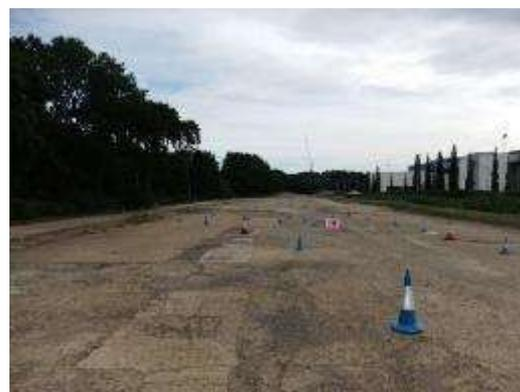
Fig 5.41 - Further surface degradation, patch repairs and scars of previous uses on the track towards the southern end of the Railway Straight.
