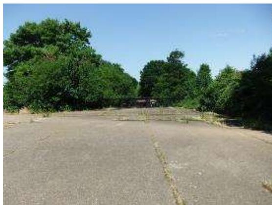
Fig 5.72 - Race track surface laid over the Cobham Bridge.
