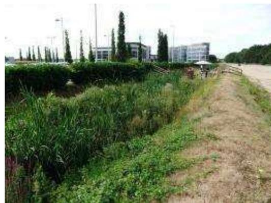
Fig 5.53 - Wide drainage channel, constructed c.2005 alongside the eastern edge of the Railway Straight, as part of the flood alleviation measures for the northern end of the Brooklands site.
