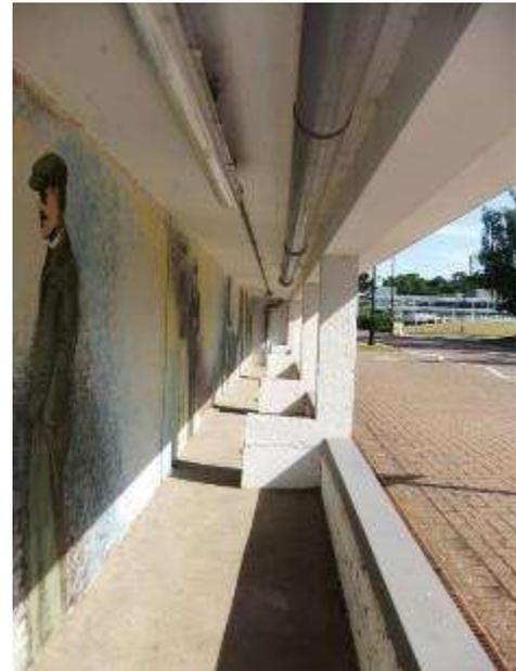
Fig 5.62 – Raised floor levels evident along with remains of former pit divisions and enclosures. 'Modern' in-fill wall (left hand side) decorated with motor racing mural.
