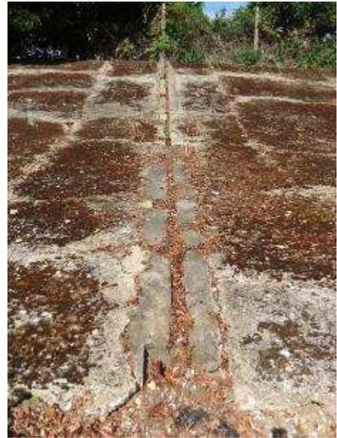
Fig 5.114 - Scar running through track, indicative of a former fence line with post holes to the left of the main groove cast through the surface.
