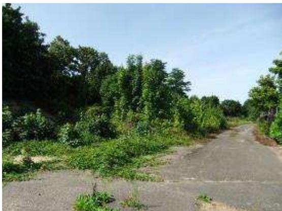
Fig 5.107 - Dense vegetation and tree growth established across the track surface. Condition and extent of any further historic remains within this area are unknown.
