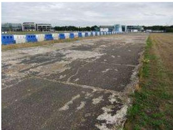
Fig 5.46 - Remains of tarmac top coat to surface of ‘Sahara Straight’ and erosion to track bays along their outer edges.
