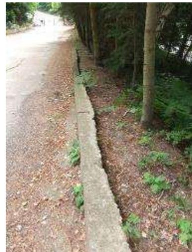
Fig 5.19 – Low-level in-situ cast concrete kerbing to the south-western edge of Dunlop’s Delight.
