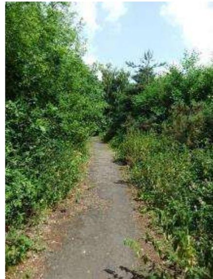
Fig 5.84 - Encroaching vegetation along the sides of the Aerodrome Road, leading to the loss of the edges and making its alignment difficult to distinguish.
