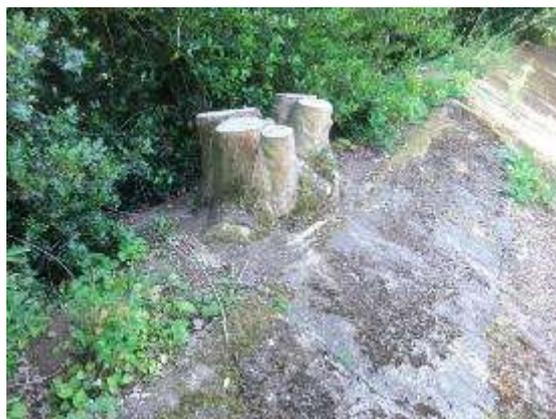
Fig 5.76 - Tree growth adjacent to the upper track edge has damaged the track surface, with localised concrete repairs clearly evident.
