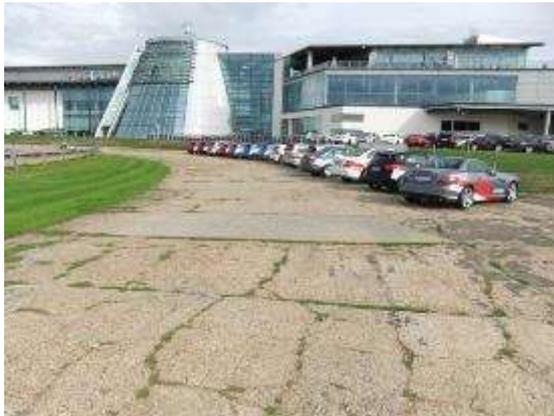
Fig 5.44 - Various degrees of surface degradation to the track, including some tarmac surfacing and modern patch repairs.
