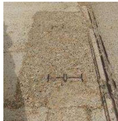
Fig 5.39- Remains of a Bellman hangar T184, including the metal channels for the sliding doors and metal columns now cut off flush with the raised concrete floor (laid over the former race track).
