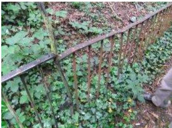
Fig 5.79 - Tops of railings removed as the result of Health & Safety concerns, exacerbating further corrosion and causing scarring to the top rail.
