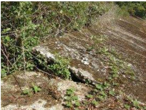
Fig 5.115 - Areas of collapse and undermining to the top edge of the banked track.
