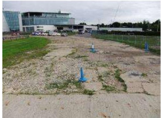
Fig 5.45 – Significant surface degradation to the northern end of the ‘Sahara Straight’. Inappropriate replacement concrete bay in the foreground.
