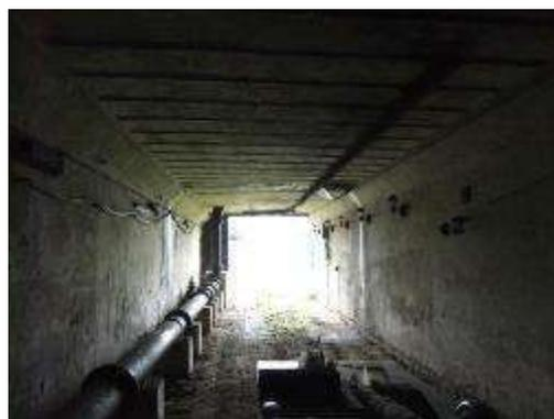
Fig 5.9 – World War 2 alterations to interior of the Competitors' Tunnel evident to the lowering and reinforcement of the ceiling.
