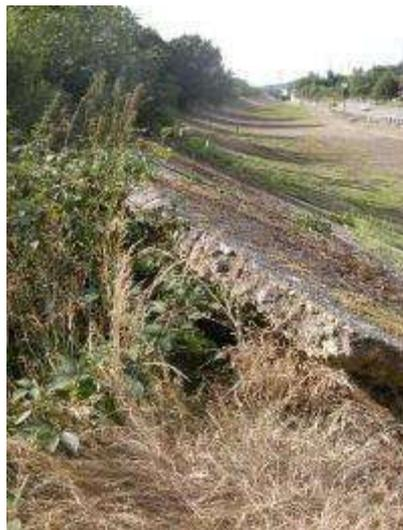
Fig 5.101 - Significant areas of undermining to the top edge of the race track as a result of burrowing animals.
