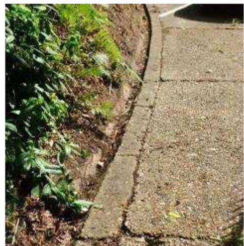
Fig 5.55 – The inner gully detail and concrete bays forming the surface of the Campbell Circuit Banking Bend.
