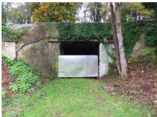
Fig 5.8 – Southern entrance to the Competitors' Tunnel, structural movement evident on left hand side.
