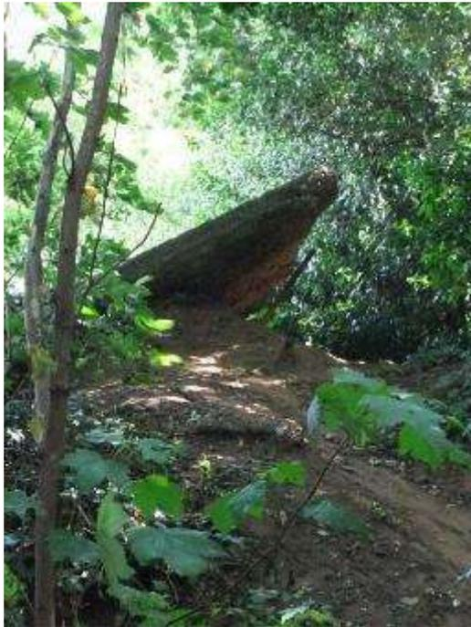
Fig 5.77 - Unsupported upper section of Byfleet Banking (southern end) following the erosion and washing away of the support banking below.
